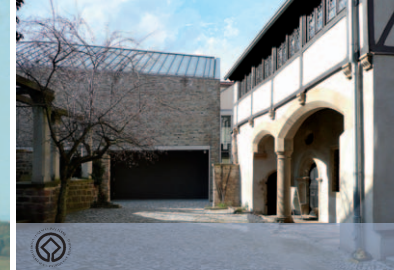
Luthergeburtshausensemble in Lutherstadt Eisleben, Architekturpreis des Landes Sachsen-Anhalt 2007 The Luther's Birthplace Ensemble in Lutherstadt Eisleben, Architecture Award of the State of Saxony-Anhalt 2007
